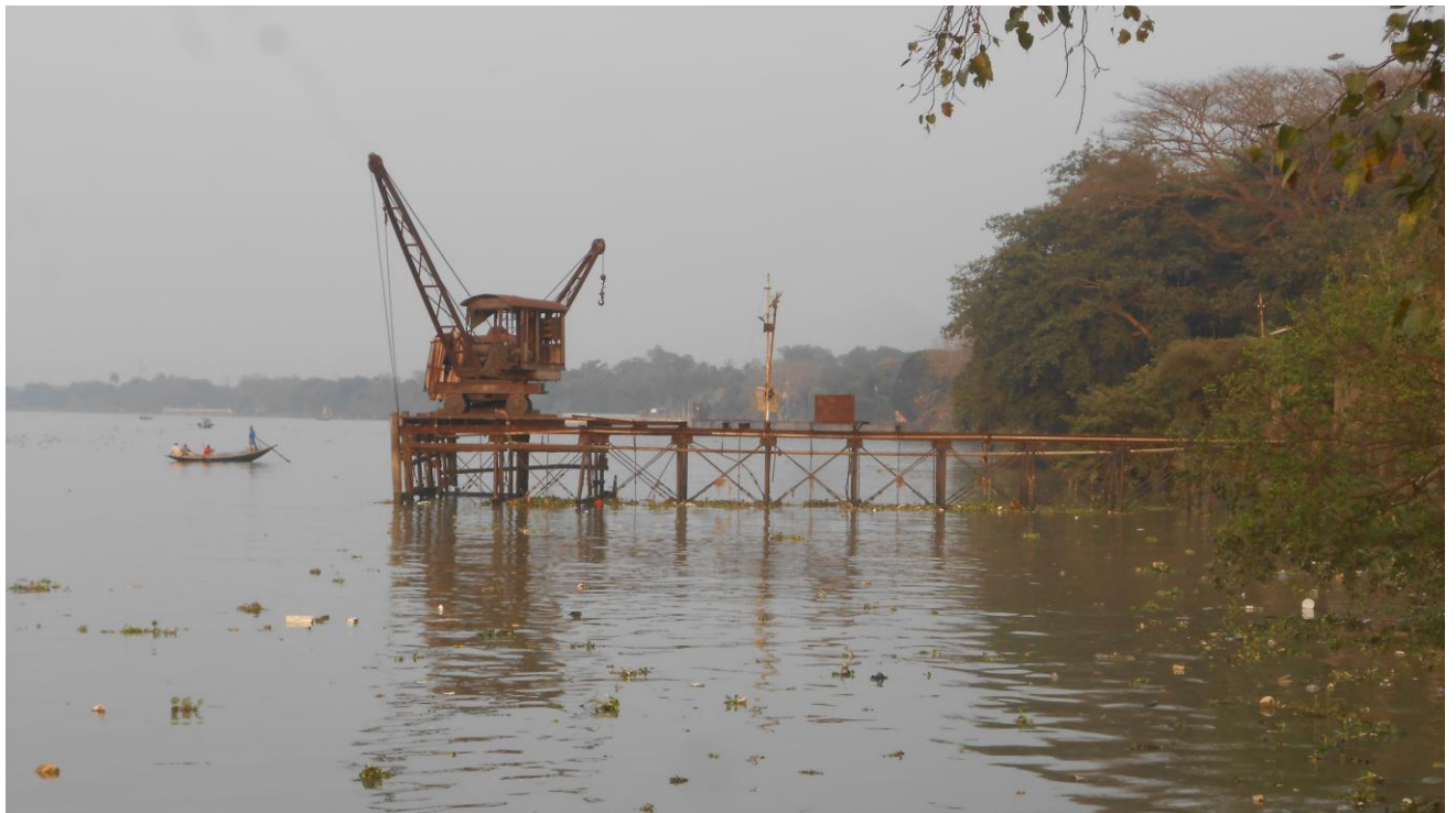
Plate 106 – Water Pumping Station , Budge Budge , 22°29'25.80"N 88°10'56.69"E
