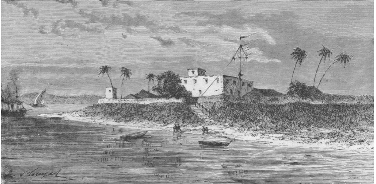
Plate 8 – Diamond Harbour , Chingrikhali Fort
